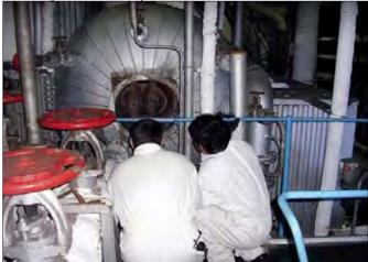
a little longer. However, he agreed to stop the circulation and pumped the mixture into a shore-side bowser. In the meantime, he asked the prime repair contractor to arrange for the door of the starboard boiler steam drum to be opened so that the internal surfaces of the boiler could be inspected.
