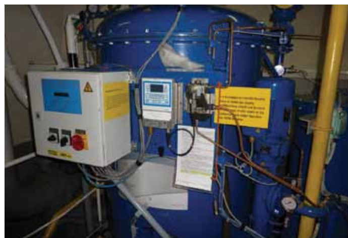
^ Oily water separator (OWS)
