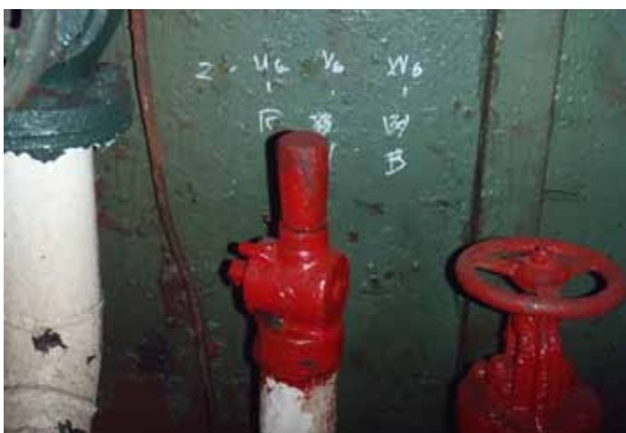
^ Screw cap replaced by wooden plug
