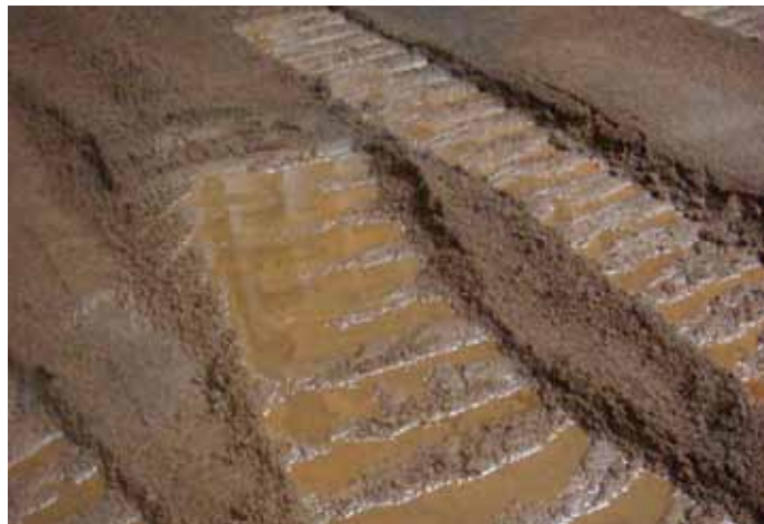
^ Water seen in the tracks of a bulldozer during trimming of sinter feed ore at Santana, Brazil
