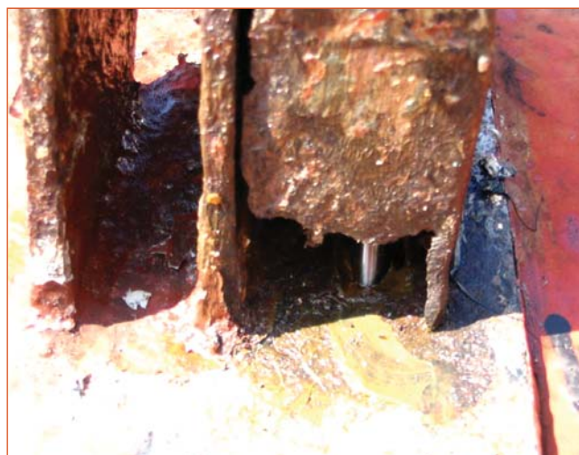
CORROSION AND WASTAGE
