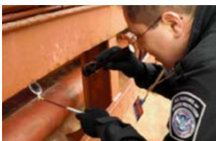
1 INSPECT ALL SURFACES
