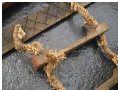
TOP PART OF THE LADDER DAMAGED
