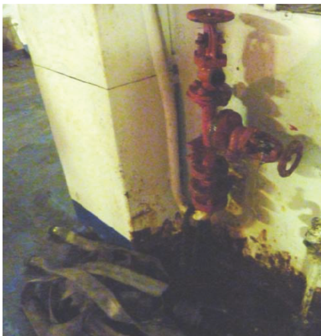
A ship with poorly maintained fire-fighting equipment indicates amongst other things that the safety management system is not working.
