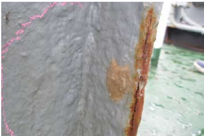
^ On safety rails and supports
