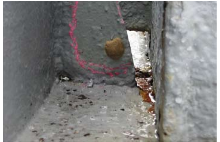
^ On hatch covers and coamings
