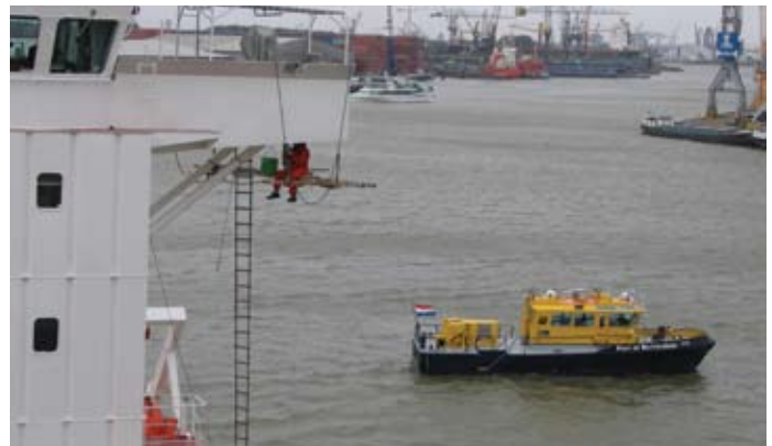
^ Portable ladders should not be used as a stage or a suspended platform to work from
