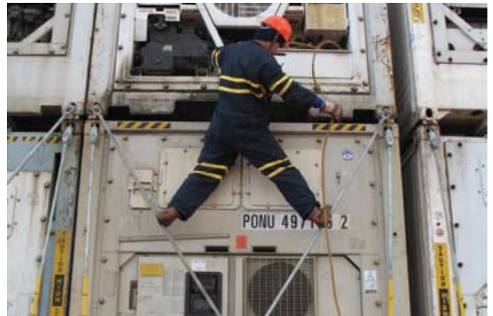
^ Dangerous act of working aloft. No safety harness or portable ladder present. This is not a safe practice
