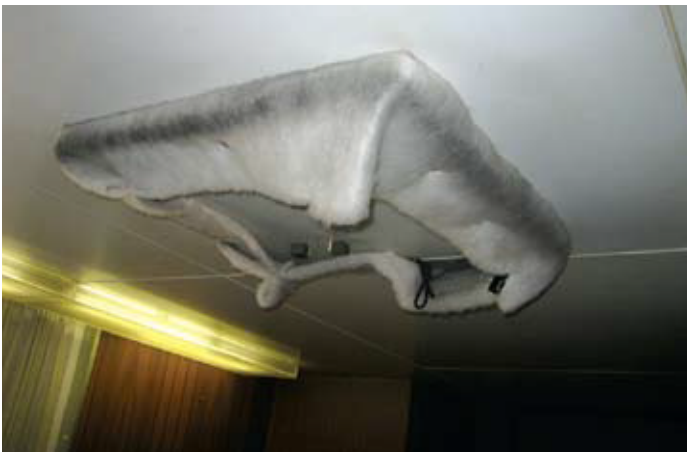
^ Ventilation and heating – Poor standard of ventilation and air movement resulting from unacceptable alterations
