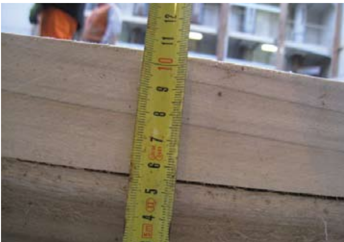
^Dunnage used should be adequate depth
