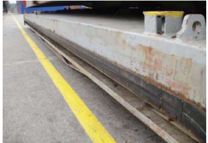
^ Hatch cover longitudinal joints such as these would have to be in good condition to prevent water ingress
