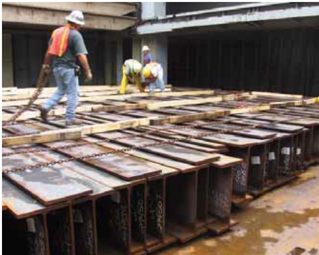
First tier of nested I-Beams stowed in the hatch square. Tightly stowed I-Beams are secured with chains to deck fittings.
