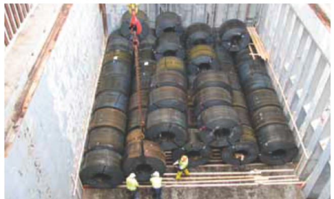
Coils dropped straight into the hatch square. Note use of wire ribbon slings.
