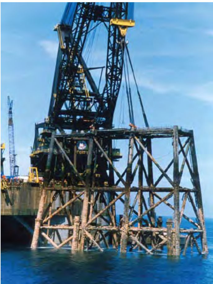
Removal of a jacket
