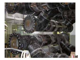
Figure 27: Glass reinforced epoxy pipe construction Courtesy NOV Fiber Glass Systems
