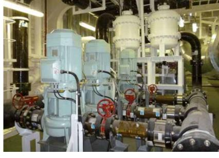
Figure 26: Open loop system washwater treatment plant (Hydrocyclones (white) in background)
