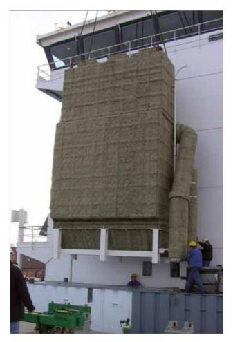
Figure 51: Installation of a Couple Systems dry exhaust gas cleaning unit
