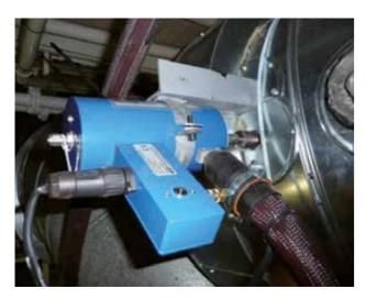
Figure 44: Heated sample line and probe for extractive analyser
