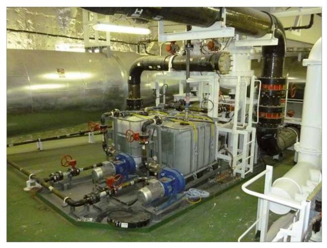
Figure 47: Washwater treatment residue collection
