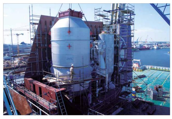
Figure 41: Alfa Laval's trial EGC unit during installation Courtesy Alfa Laval
