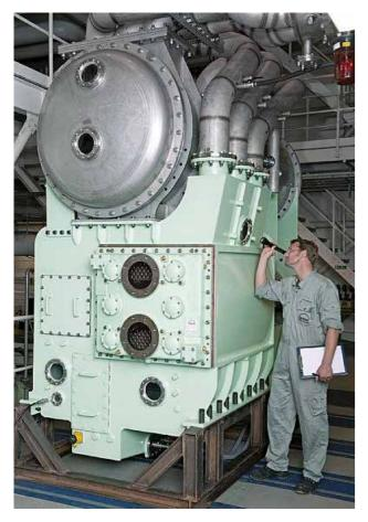
Figure 39: EGR system high-pressure scrubber unit Courtesy MAN Diesel & Turbo
