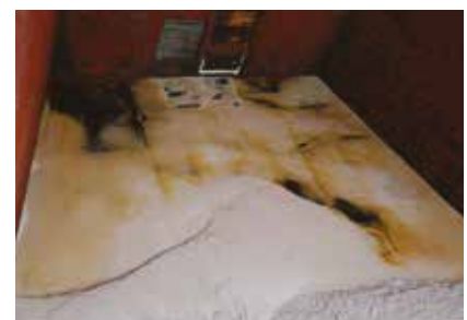
Water ingress via a faulty bilge valve will cause cargo damage
