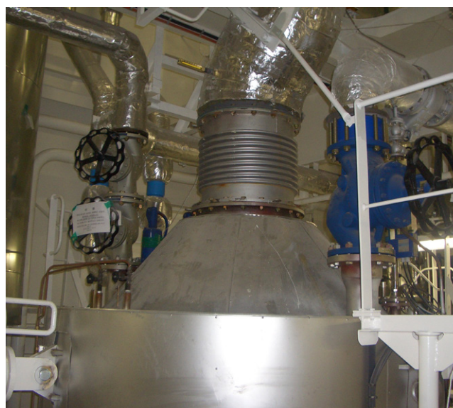
Figure 14: Exhaust pipe compensators (bellows)
