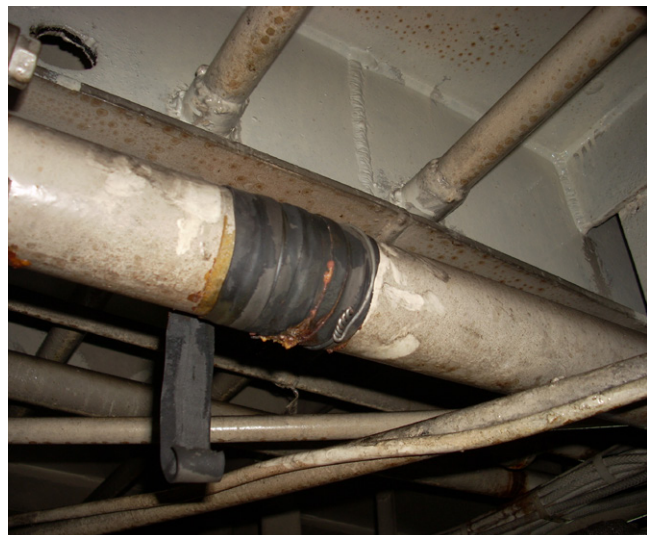
Figure 9: Temporary pipe repair
