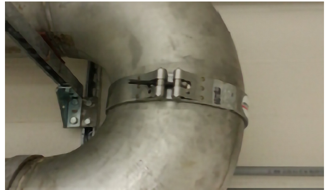
Figure 17: Rubber insertion and hose clip
