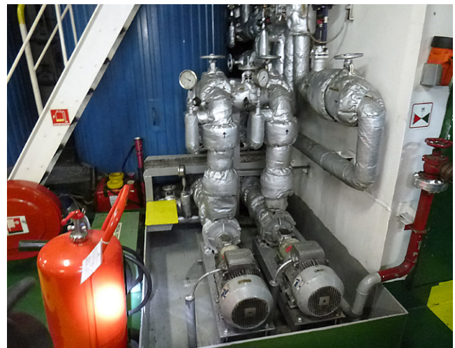
Figure 10: Typical steam piping
