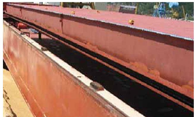
Figure 10: Compression bar and drain channel in good condition
