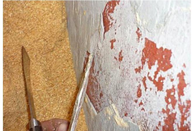
Figure 6: Surveyor scraping cement from the bulkhead in the hold
