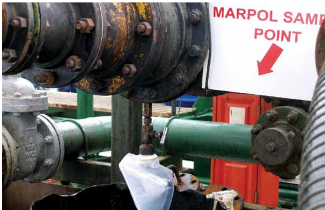
^ MARPOL sample point showing cubitainer attached
