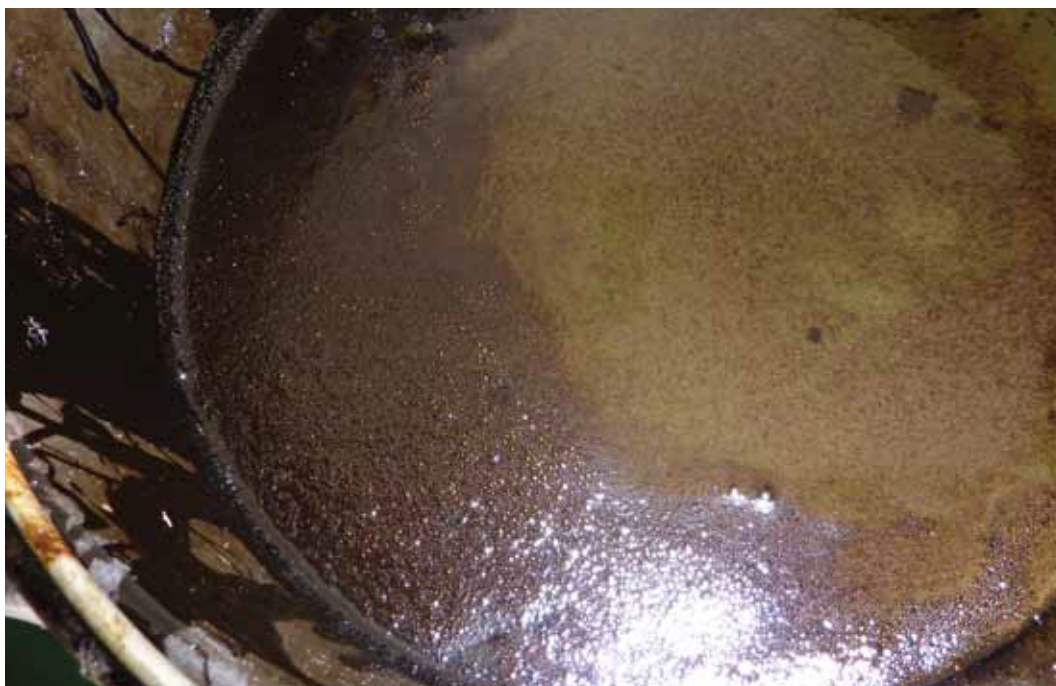
^ Check bunkers for signs of frothing
